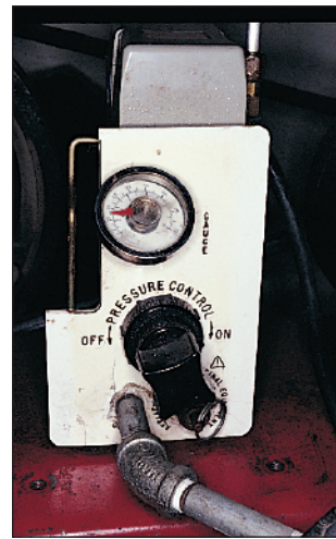
This particular air compressor has a built-in pressure regulator. The pressure control on the panel selects the regulated pressure. The gauge on the panel reads regulated pressure not the tank pressure. If you use an air grinder, whatever compressed air source you use should have an adjustable regulator.
